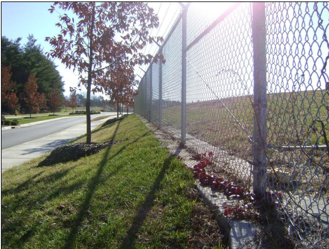
Figure 2-12 – Airport Perimeter Fence
