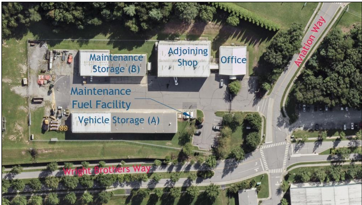
Figure 2-13 – Airport Maintenance Facilities
