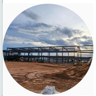
Work is quickly progressing on the new north concourse. Steel work is moving along quickly, and horizontal steel work for the vertical decking is now taking place. The framework for the north concourse is expected to be completed in March!
